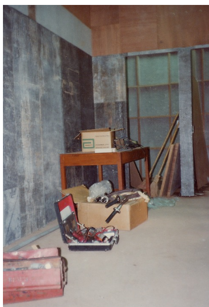
Figure 7. Construction of the radiography room ; three refugee helpers and I constructed many lead plates for the radiography room ourselves.
